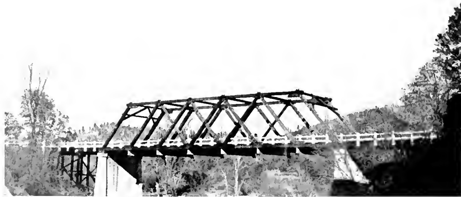
Completed job with new truss in place and falsework removed
